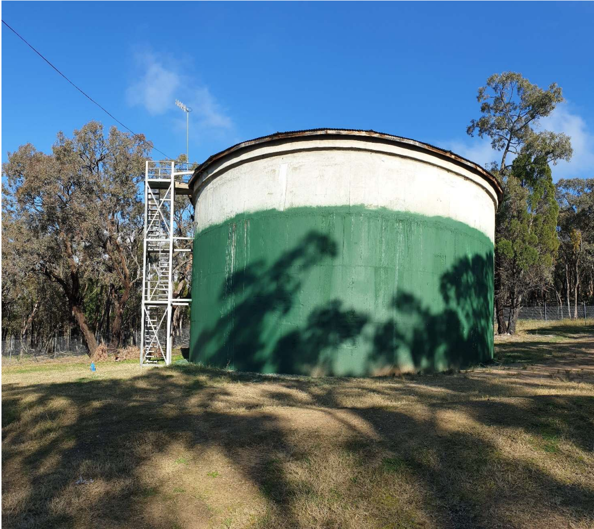
Figure 5-5 Martin St reservoir
